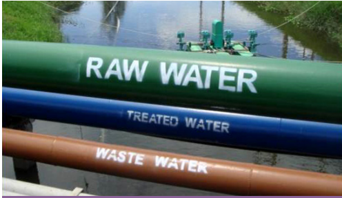
At Amata, pipes run separately for each type of water. 70% of wastewater is reclaimed by RO membrane systems and supplied to factories, while the remaining 30% is used for green areas.
